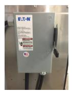
**Electrical Service Disconnection (High Voltage):** The source of power for the VBX-160. To disconnect power from the VBX-160, move the lever to the OFF position.
